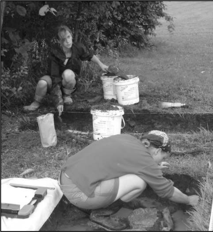
Figure 5 – Excavation of blacksmith shop foundation walls, brick from the forge and a floor ‘sleeper’ trench after one of the numerous deluges that plagued the summer season.
